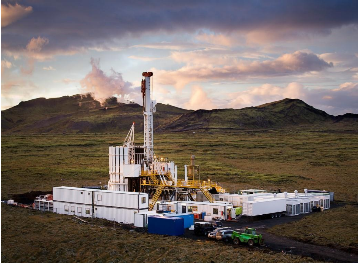
Slika 4-2. Bušaće postrojenje Tyr Drillmec HH-300 ( https://www.jardboranir.is/equipment-rigs/tyr/ )
