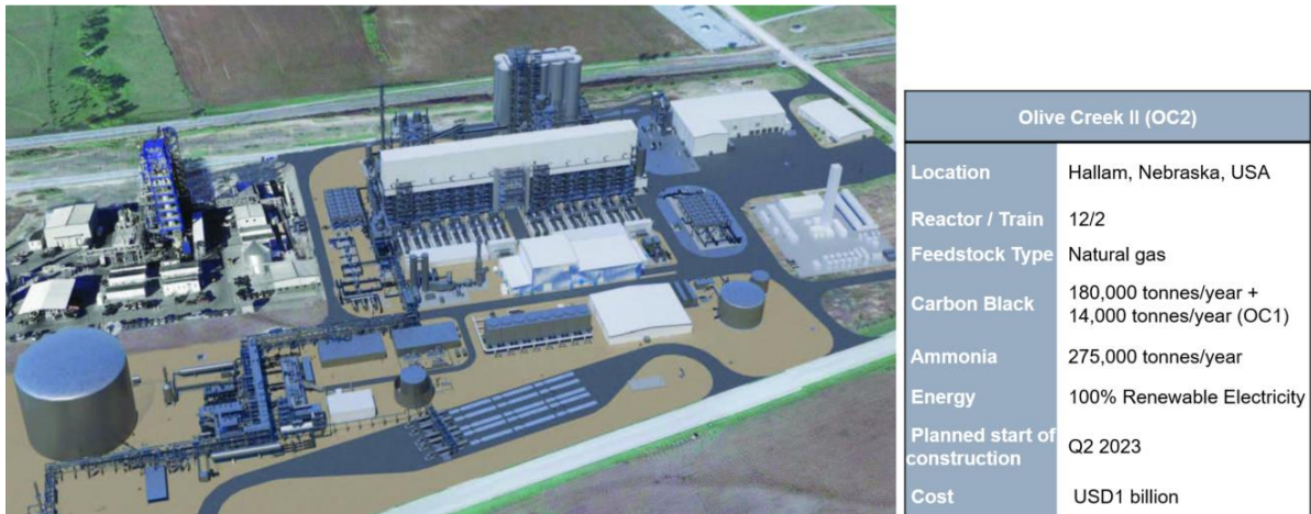
Figure 5-14. Monolith’s Olive Creek II (OC2) design concept (left) and project summary (right) (after Mesrobian, 2022).
