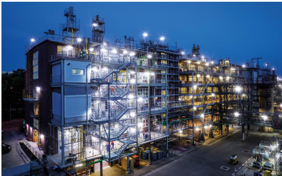
Figure 5-2. BASF methane pyrolysis test facility in Ludwigshafen, Germany (BASF, 2021c).
