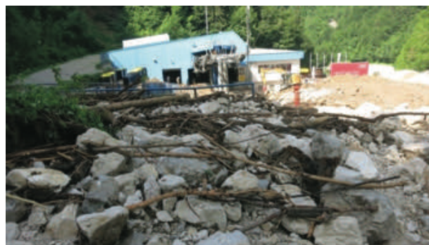
Figure 1 The Krvavec bottom station of the cabin lift after May 2018 event.
