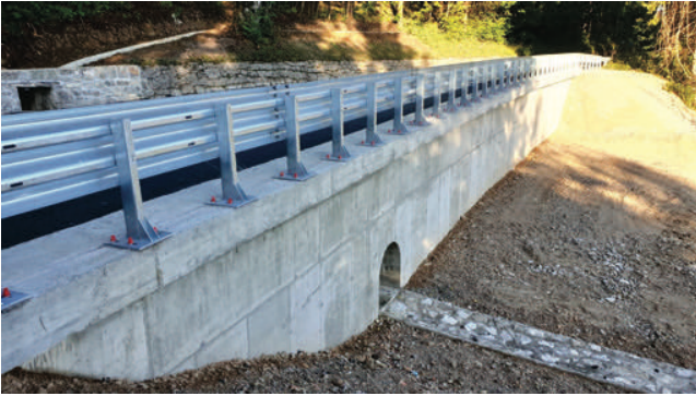
Figure 7 Dedin landslide on state road DC3 (section 015) at km 2+060 after remediation works.
