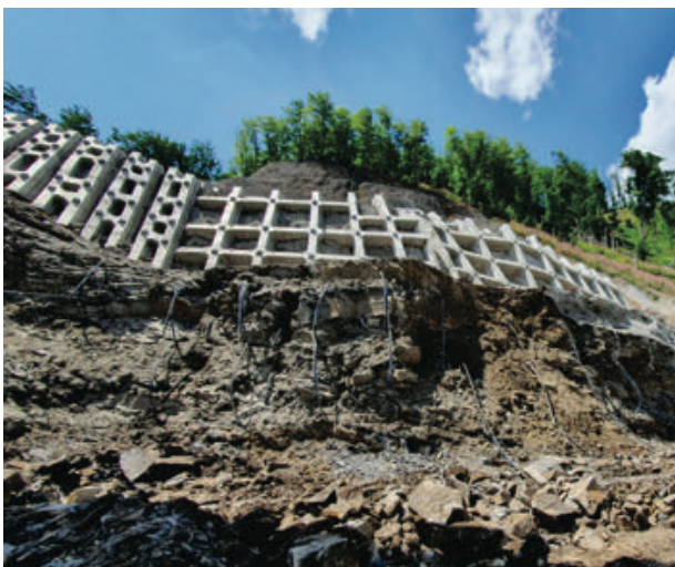
Figure 7 Photo of remediation measures.
