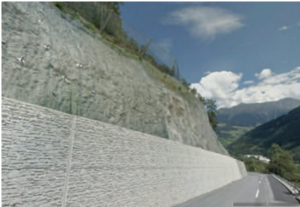
Figure 19 Serfauserstrasse as seen from the road (Google Earth Pro, 2018).
