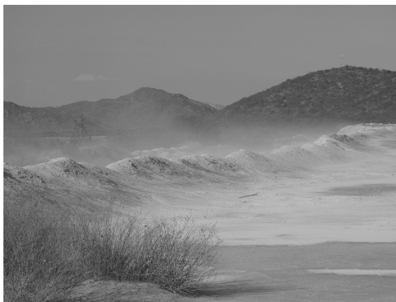
Figure 14: The tailings dam wind erosion (Kombat, Namibia) [48].
