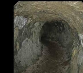
**Excavation** was performed by underground mining, shafts still carries the traces of blasting.
