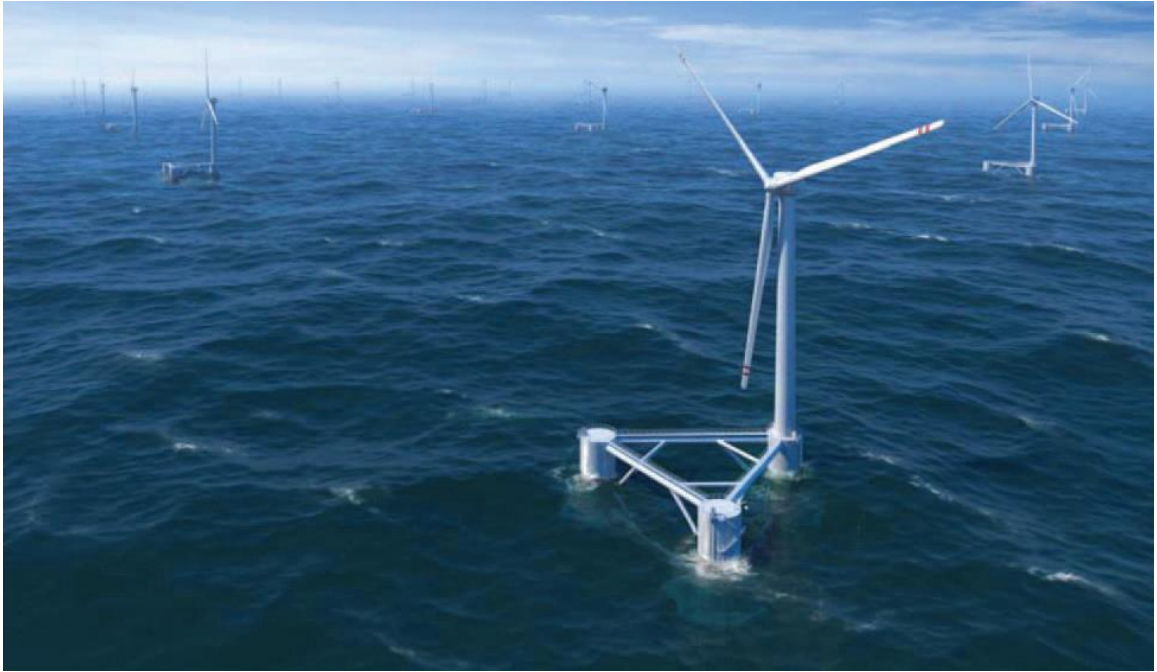
Slika 4-11. Principle Power tip poluuronjive turbine (Principle Power)
