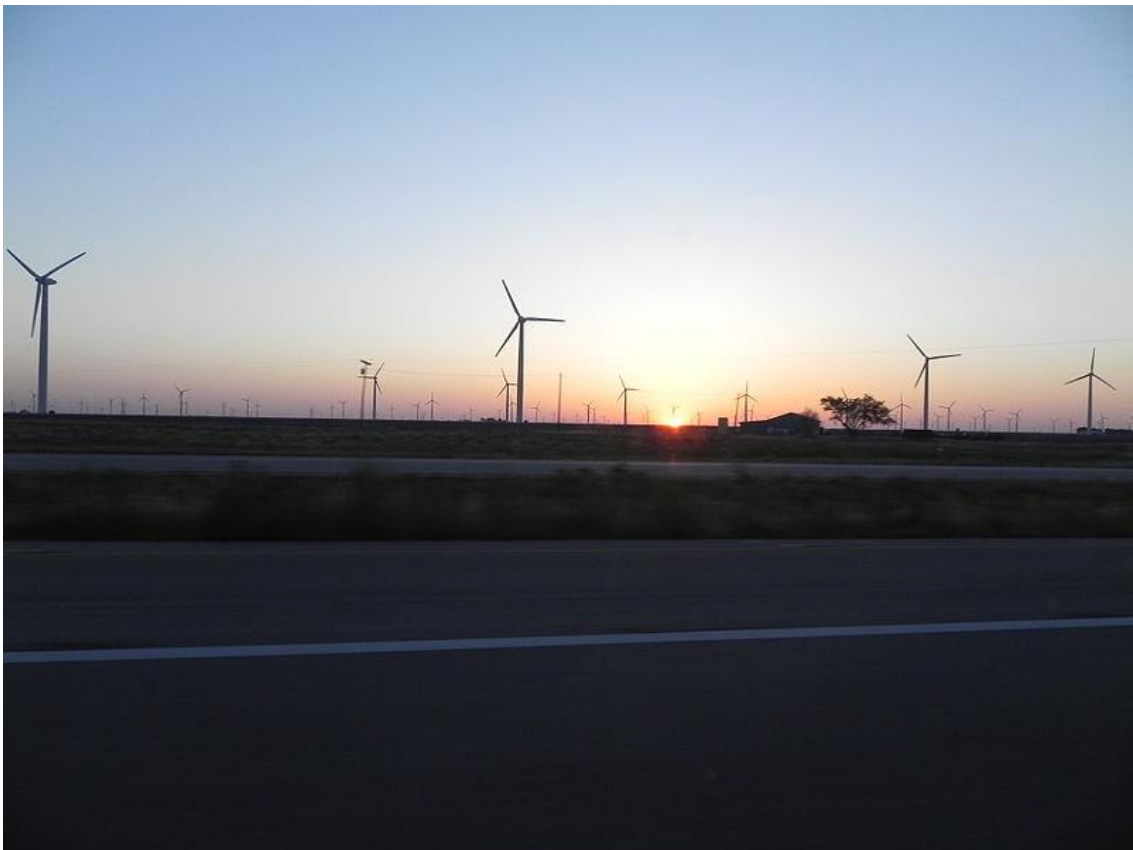
Slika 4-1. Roscoe vjetroeletktrana (Power Technology)
