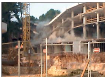
Slika 4.8. Miniranje dilatacije jug. Figure 4.8. Blasting of the southern wing.
