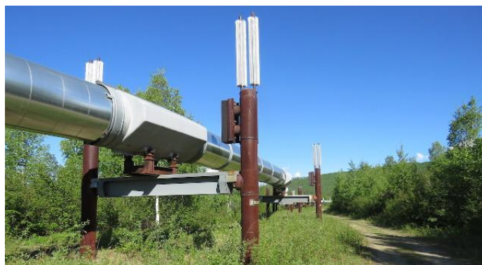
Slika 3-5. Nosaci cjevovoda ( https://www.oilandgaseng.com/ , 2020)
