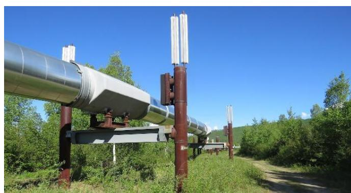
**Slika 3-5.** Nosači cjevovoda (<https://www.oilandgaseng.com/>, 2020)
