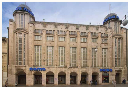
The front entrance to the NAMA department store / Prednji ulaz u zgradu NAME
