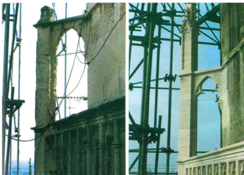
Figure 2-3. Pinnacle before and after the restoration (Crnković, 1994)
