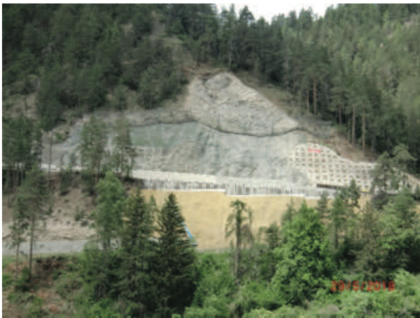
Figure 20 Serfauserstrasse stabilised slope, with a rockfall barrier at the top, anchored high-tensile steel mesh in the middle and greening mats in the bottom part of the slope.
