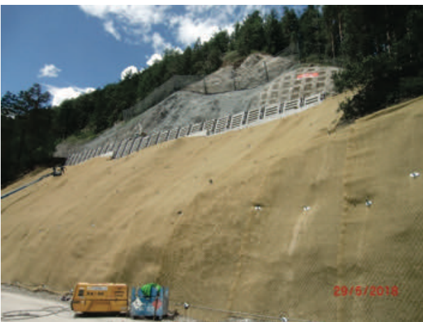
Figure 15 Final works underway at the Serfauserstrasse, with a highlight on the greening mat along the bottom part of the road.
