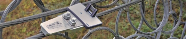
Figure 6 Example of the Geobrug Guard installation (Geobrugg 2022b).
