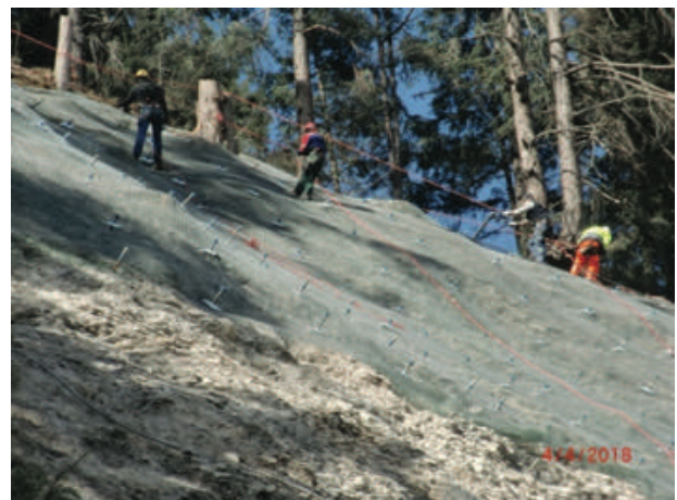
Figure 11 Rope access work while installing the high-tensile steel mesh.
