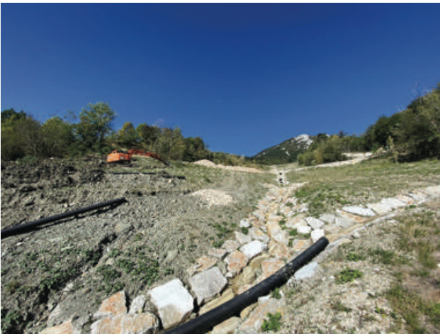
Figure 8 Excavating work on the landslide in October 2021.
