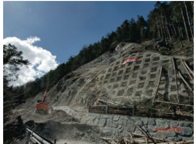
Figure 8 View of the beginning of works to clear the road from the landslide mass.
