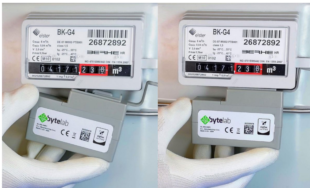
Fig. 2. Installation of module for remote reading of natural gas consumption (Šimić, 2020).
