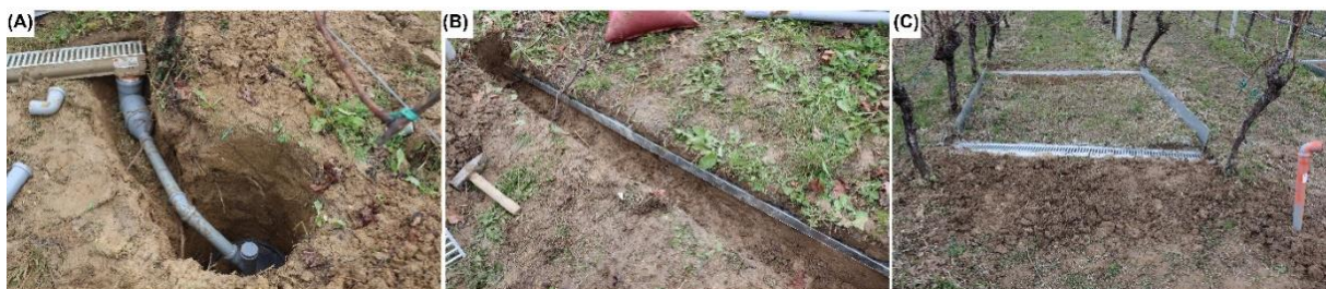
Figure 4. Process of installation of surface runoff collection instruments: (A) collection tank placement and pipe connection, (B) flow guide placement (C) border and drain channel placement at the SUPREHILL Critical Zone Observatory (CZO).
