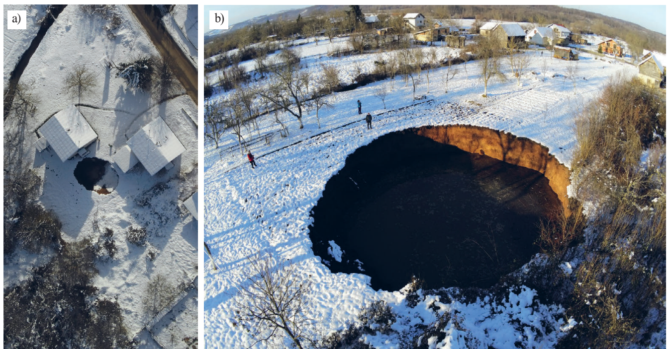
Figure 4. Dropout dolines in Mečenčani village: a) endangering adjacent houses (observation point IK31), b) the biggest doline, more than 20m in diameter and about 12 m deep (observation point IK4).
