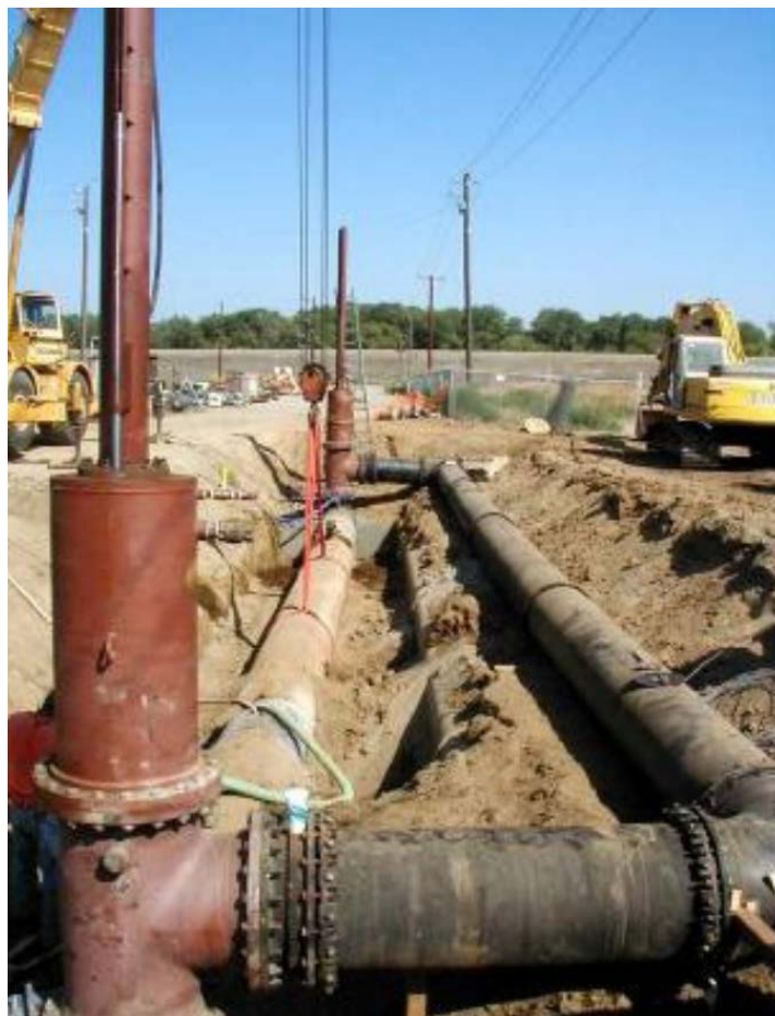
Slika 7-1. "Hot tapping" (www.hottap.com, 2016)
