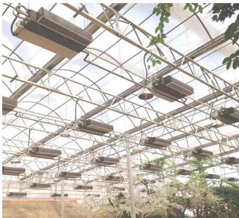
**Slika 6-3.** Stropni ventilokonvektor (Jindun Equipment, 2020)
