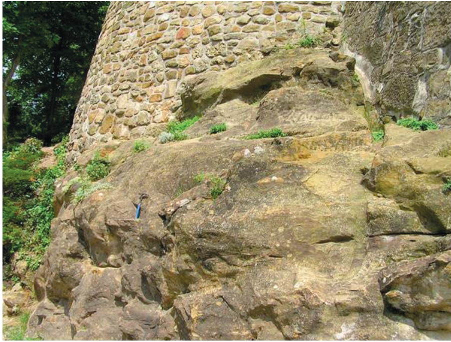
Figure 22. The walls of the Trakošćan Castle built on natural foundations composed of bedded conglomerates and sandstones (photo by R. Avanić).
