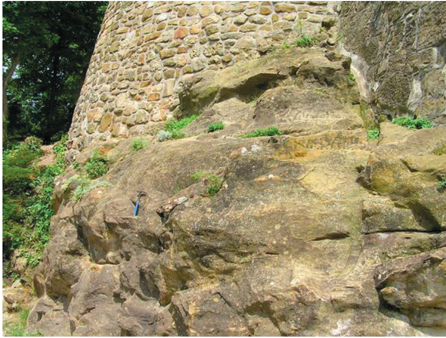
Figure 22. The walls of the Trakošćan Castle built on natural foundations composed of bedded conglomerates and sandstones (photo by R. Avanić).
