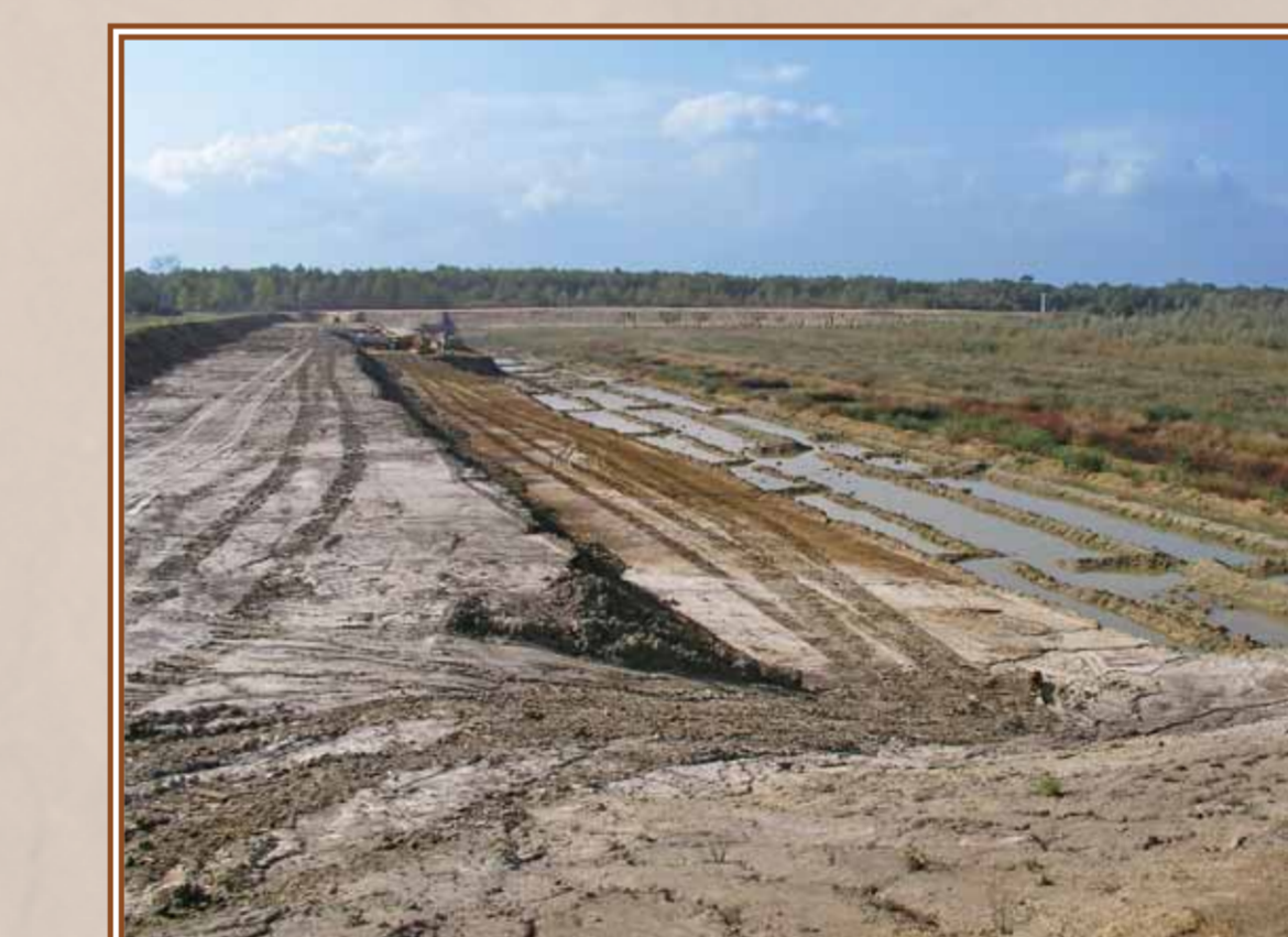
Brick clay open-pit Retica
