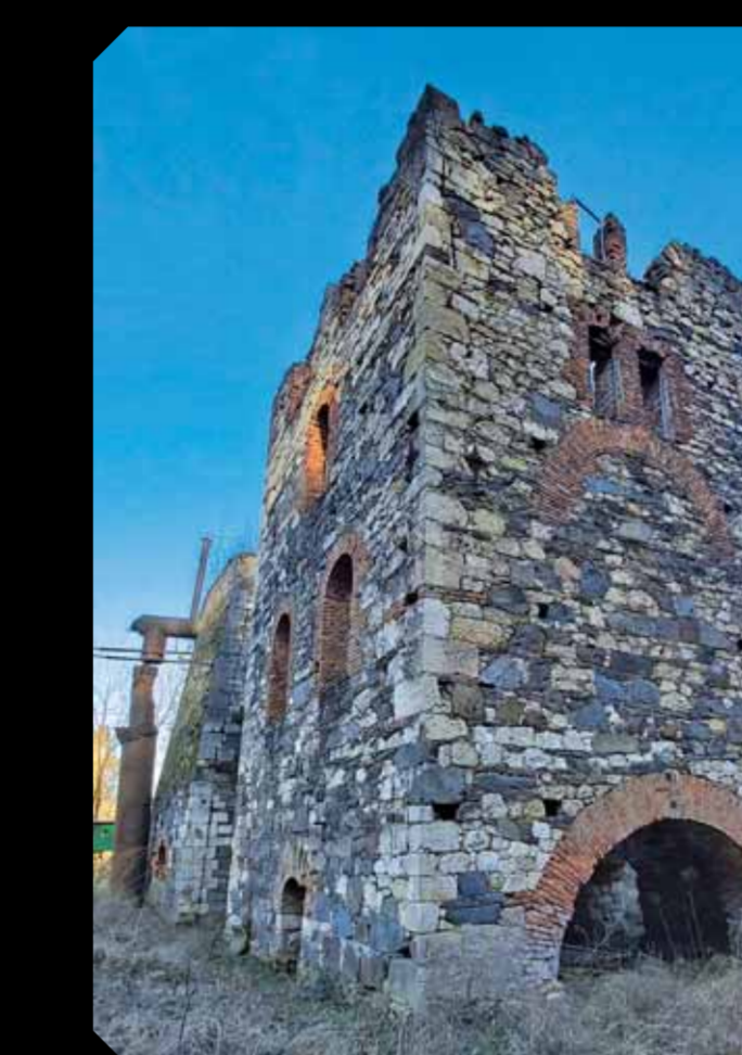
The Bešlinac blast furnace - the state of art of its time
