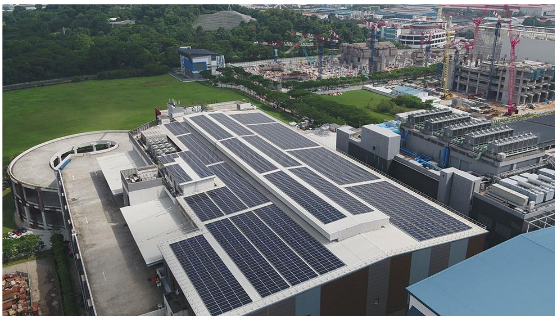
Slika 3-6. Solarni paneli na krovu Green Hub-a (Bollore Logistics)
