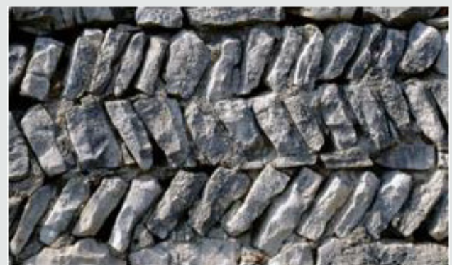
Figure 3: Side walls of the St Barbara Church built in the "fishbone" style (Photo by N. Fazinić).
