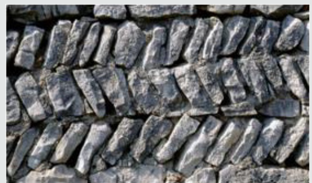
Figure 3: Side walls of the St Barbara Church built in the "fishbone" style (Photo by N. Fazinić).
