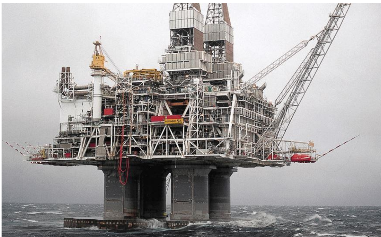
Slika 4-1. Platforma Hibernia (mwws.nl, 2020)
