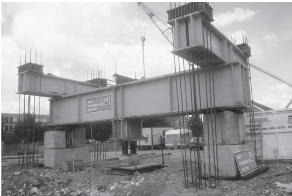
Slika 5-1 Statičko ispitivanje pilota (Cementation Piling and Foundations Ltd., Rickmansworth)
