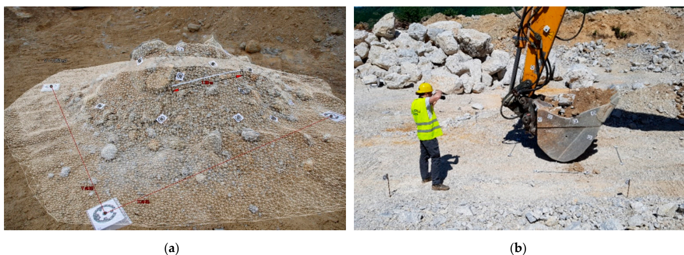
Figure 2. (a) Measuring volume of the bucket load and (b) angle of repose of material.
