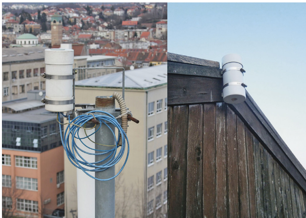
Figure 1: Left: The SQM-LE instrument at the RGN site is inside a protective box (white) mounted on the roof of the faculty building. Right: The SQM-LU-DL instrument at the Merenje site is also inside a protective box mounted on the roof of a small shed in the countryside. Both instruments have a clear zenithal area.
