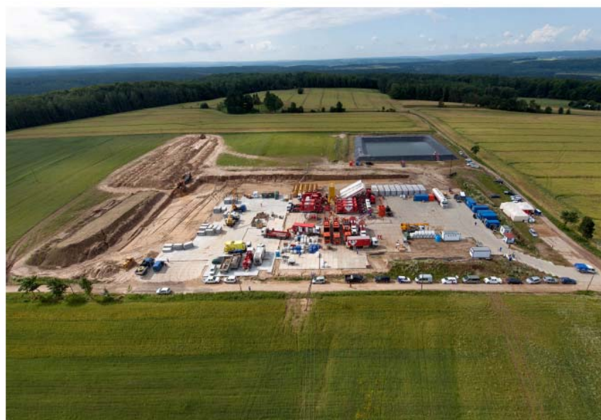
Figure 3. Well site prepared for HF.
