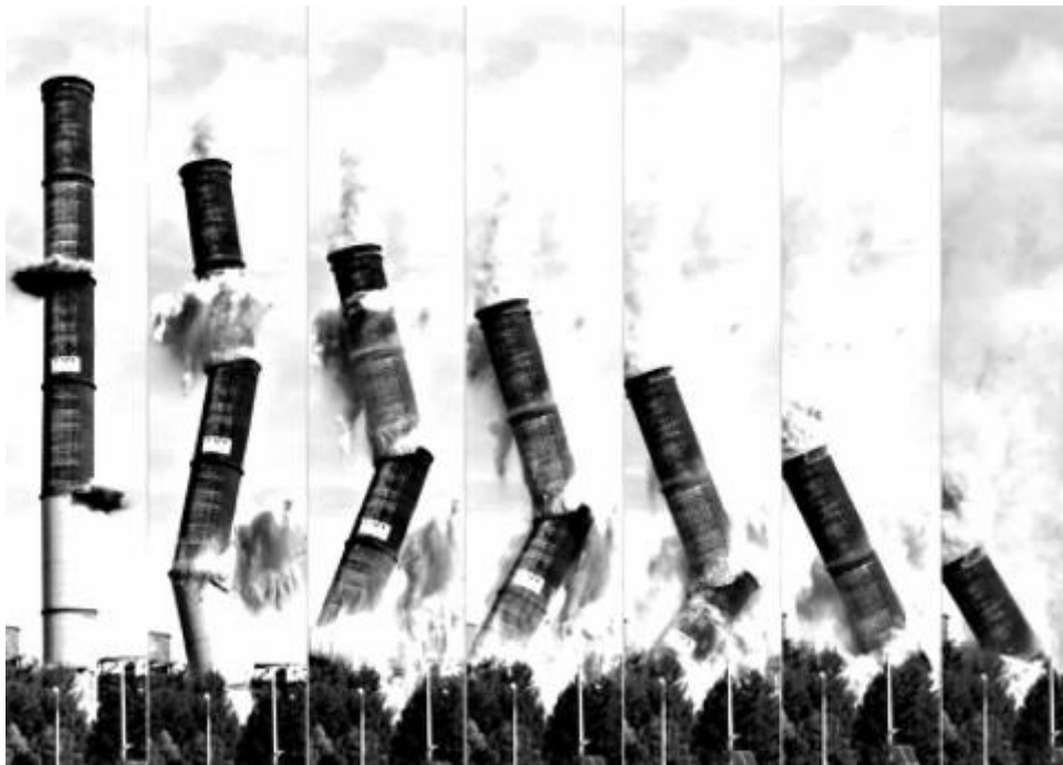
Slika 5-5 Cik-cak kolaps dimnjaka 3 ((Melzer,2015 )
