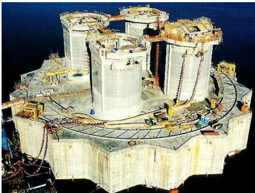
Slika 3-12. GBS postolje Hibernia platforme (Offshore Technology, 2021a)
