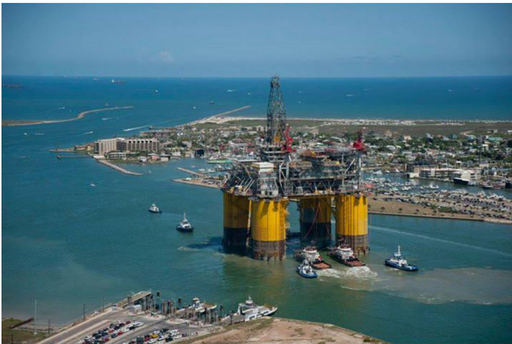
Slika 3-2. Transport platforme s nategom u nogama (hitechelectric.com)
