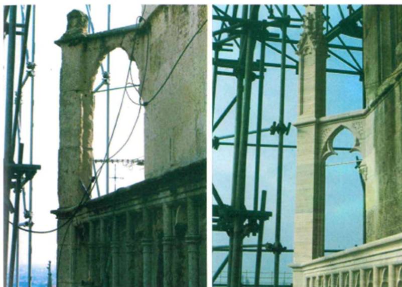
Figure 2-3. Pinnacle before and after the restoration (Crnković, 1994)
