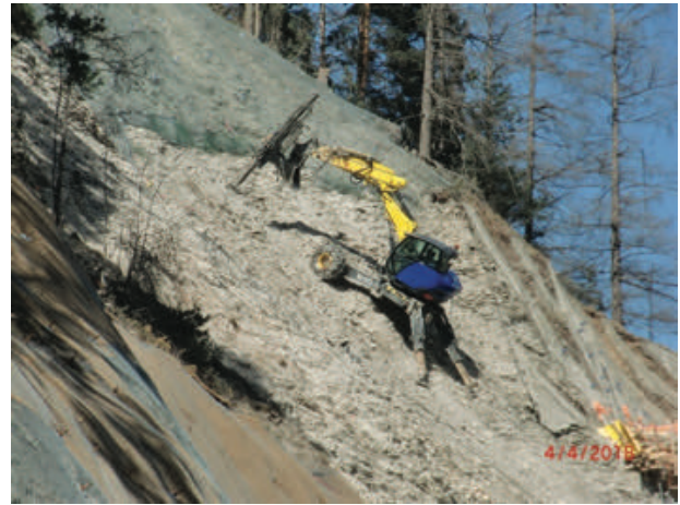
Figure 10 A walking excavator in action, drilling the next row of anchors, while being already protected from the top, as the high-tensile steel mesh is already installed.
