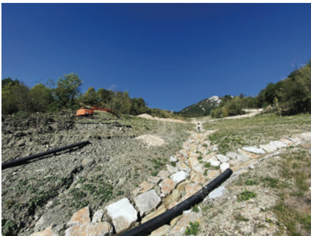
Figure 8 Excavating work on the landslide in October 2021.
