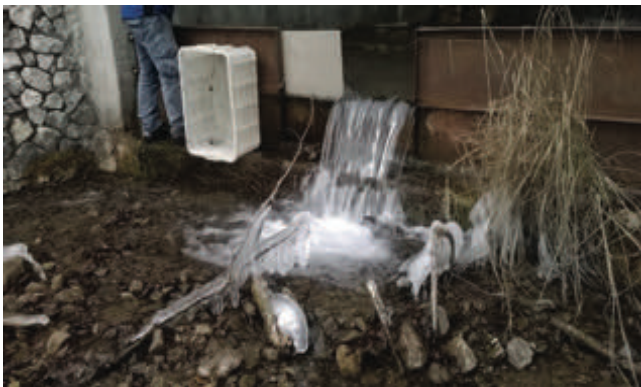
Figure 3 Thin plate weir, the hydrometer is installed behind the steel plate. Photo taken during one of the calibration campaigns.
