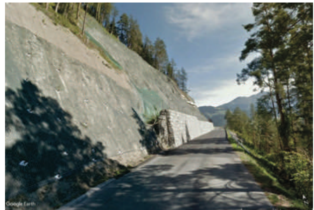
Figure 17 Ladiserstrasse as seen from the road (Google Earth Pro, 2018).
