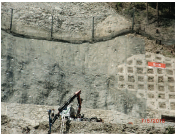
Figure 14 Drilling truck starting on the stabilisation works at the bottom part of the Serfauserstrasse instability.
