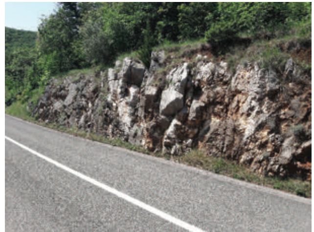
Figure 3 Example of the slope with three discontinuity sets plus random discontinuities (segment from km 16+530 to km 16+640)
