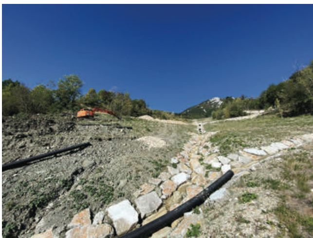
Figure 8 Excavating work on the landslide in October 2021.
