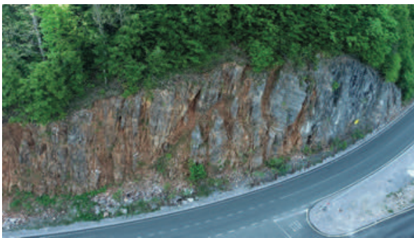
Figure 2 A view at the rock cut at the Špičunak location.
