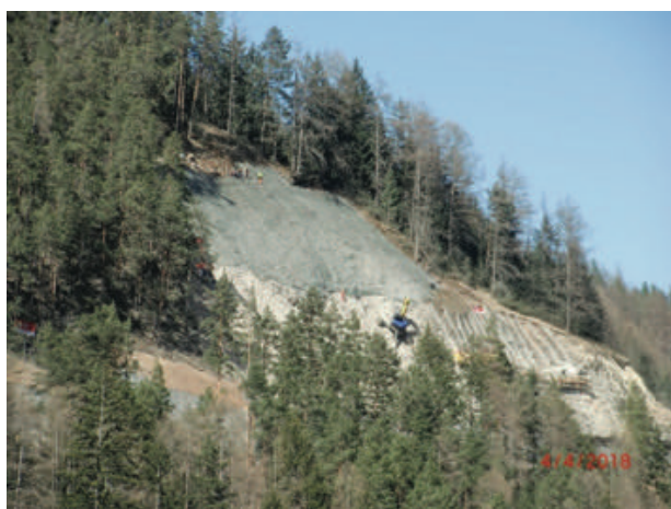
Figure 9 View of the unstable slope at Ladiserstrasse, where the first part of anchoring and mesh deployment is completed, allowing secure works underneath to be completed.
