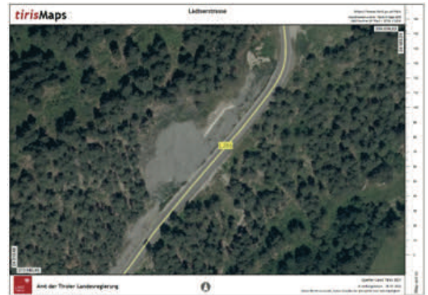
Figure 16 Orthophoto of the stabilised slope along the Ladiserstrasse (tirisiMaps, 2018).
