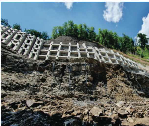
Figure 7 Photo of remediation measures.
