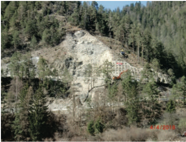
Figure 13 View of the unstable slopes along Serfauserstrasse.
