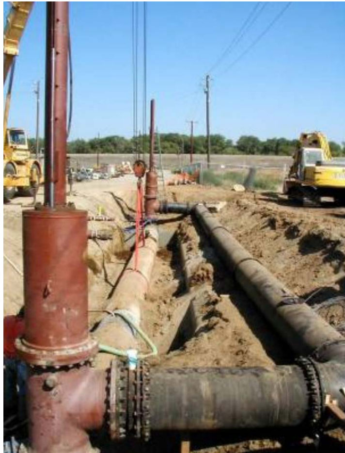
Slika 7-1. "Hot tapping" (www.hottap.com, 2016)
