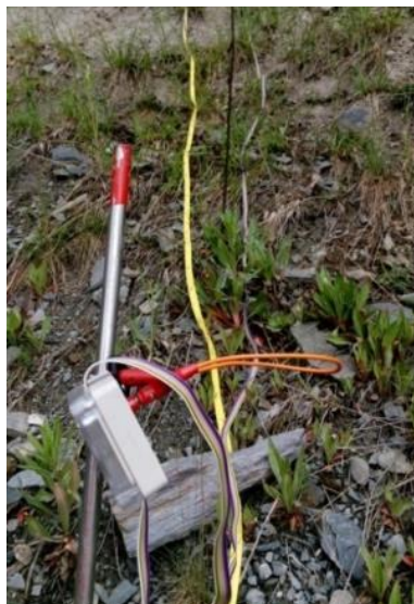
Figure 5-4 Field photo showing example of installed electrode
