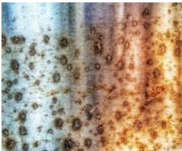
Slika 2-1. Primjer točkaste korozije (Oil and Gas Corrosion Lexicon, 2015, Himipex Oil)
