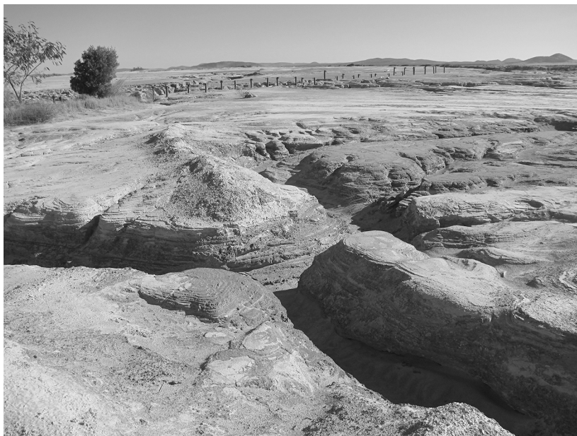
Figure 12: Unsecured and unrehabilitated tailings dam with visible water erosion (gullies) at Kombat mine in Namibia [48].
