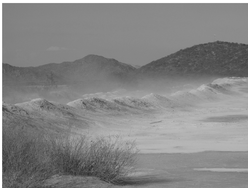
Figure 14: The tailings dam wind erosion (Kombat, Namibia) [48].
